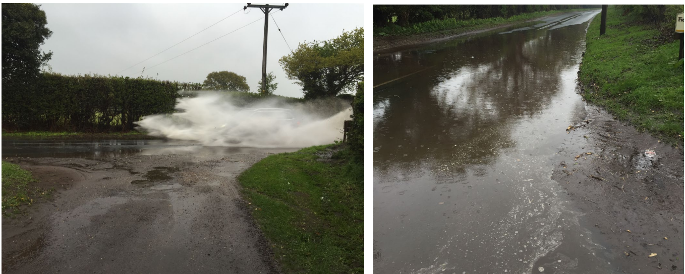
Figure 4: flooding and standing water affecting the lane and junction
